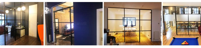
The doors themselves are a sheet of toughened glass, with bars applied front and back, using the same tape. There is no perimeter trackwork to the perimeter of the door leaf in our standard system.
